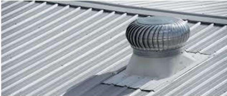
FIXING OF ROOF VENT
