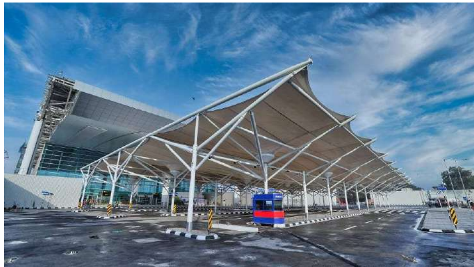
KALZIP SHEET AT IGI AIRPORT TERMINAL 3
