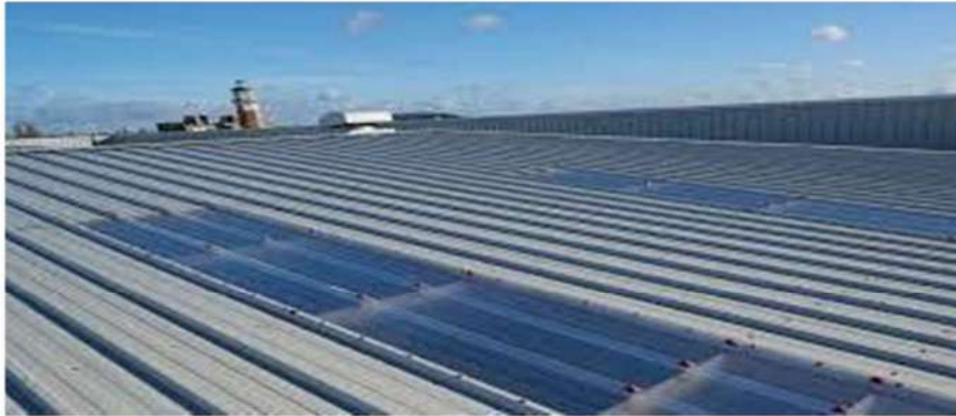
FIXING OF POLYCARBONATE
