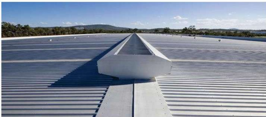
FIXING OF RIDGE VENTILATOR
